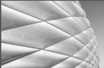
Air-inflated ETFE Cushion Facade [5]
