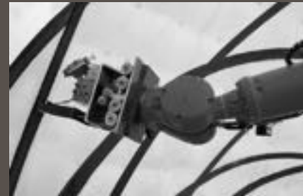
On-site robotic fibre placement [7]
