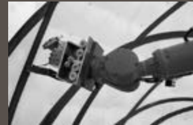
Step 2: On-site robotic fibre placement [7]
